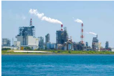
Wastewater treatment for metal-containing wastewater
